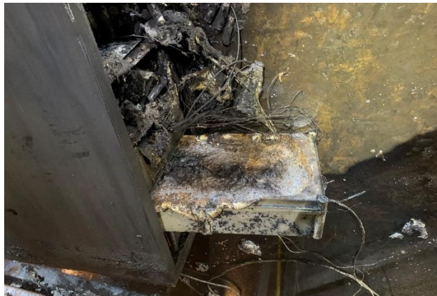
Figure 139 – Condition of InitUnitMod2 with waterline visible after Test 3.
