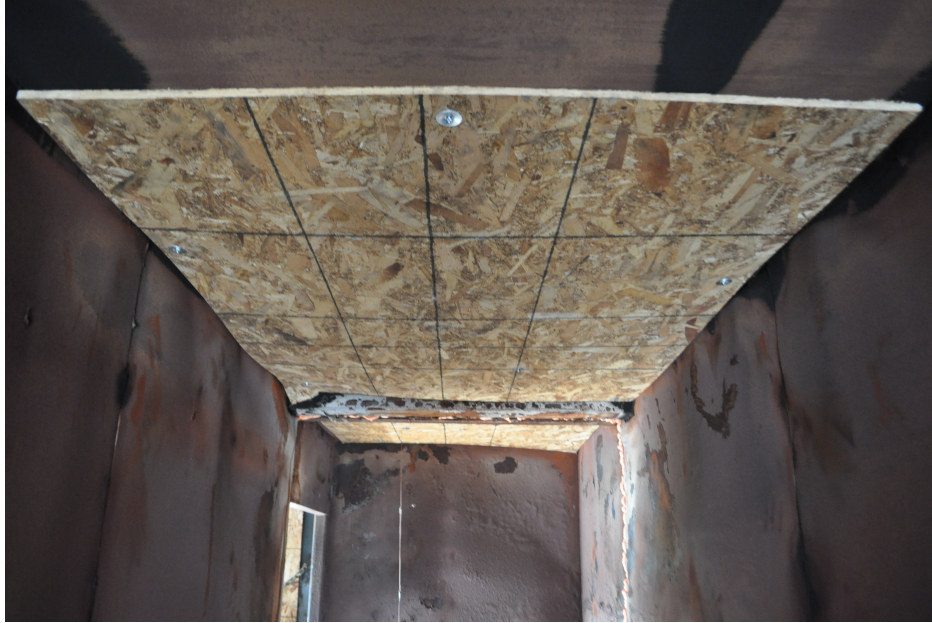
Figure 5.26: OSB on hallway ceiling for Experiment 3
